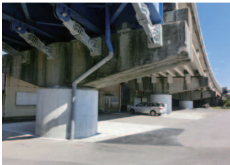
橋梁の耐震補強
