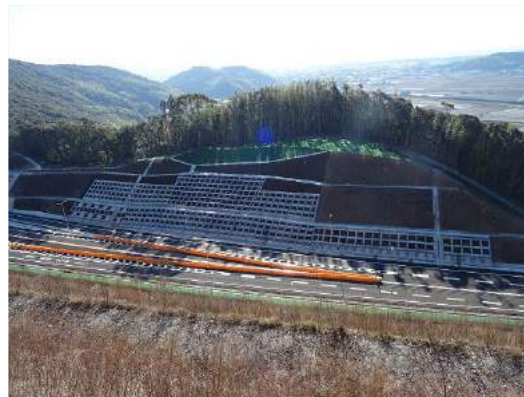
Slope disaster prevention
